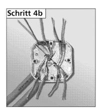
... and separate the wire pairs by colour.
