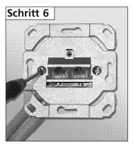
Lay on the upper housing section and tighten the locking screws until the housing is closed.
