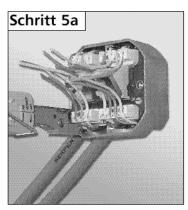
Insert the PCB in the lower housing section and connect the wires to the terminals with the LSA plus ® lay-on tool (BTR Telecom Art. No. 130 818-E).
