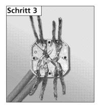
Lay in the wires in accordance with the colour coding (also see the section "Notes on connection") and the desired cable outlet direction (e.g. from the lower left).
